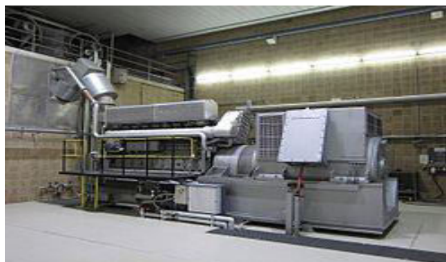
Fig:- emergency power electric generator in a water purification plant, driven by a marine propulsion diesel engine
